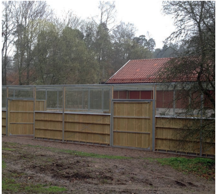
THIS COMPLEX HAS BOTH INDOOR FACILITIES AND OUTDOOR ENCLOSURES. THE EMPTY SPACE HAS OFTEN PROVED TO BE THE MOST VALUABLE ONE – THEREFORE THESE ENCLOSURES ARE ONLY USED TEMPORARILY. THEY ARE BUILT TO BE VERY FLEXIBLE FOR HOSTING DIFFERENT SPECIES AND CAN EASILY BE REMODELLED TO SUIT DIFFERENT REQUIREMENTS.
